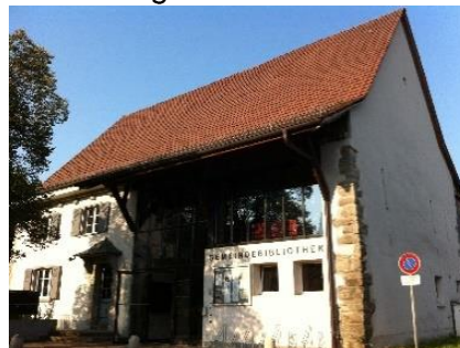
Therwil Kirchrain 2 4106 Therwil
